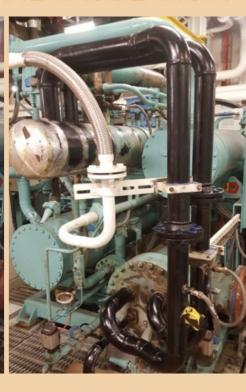
Here is an example or refitting of the piping insulation of a refrigeration facility. In order to increase as maximum as possible the piping lifetime we provide a turnkey service that includes: chipping, first painting, second painting, insulation with armaflex and then another painting over it to increase its resistance and lifetime.
